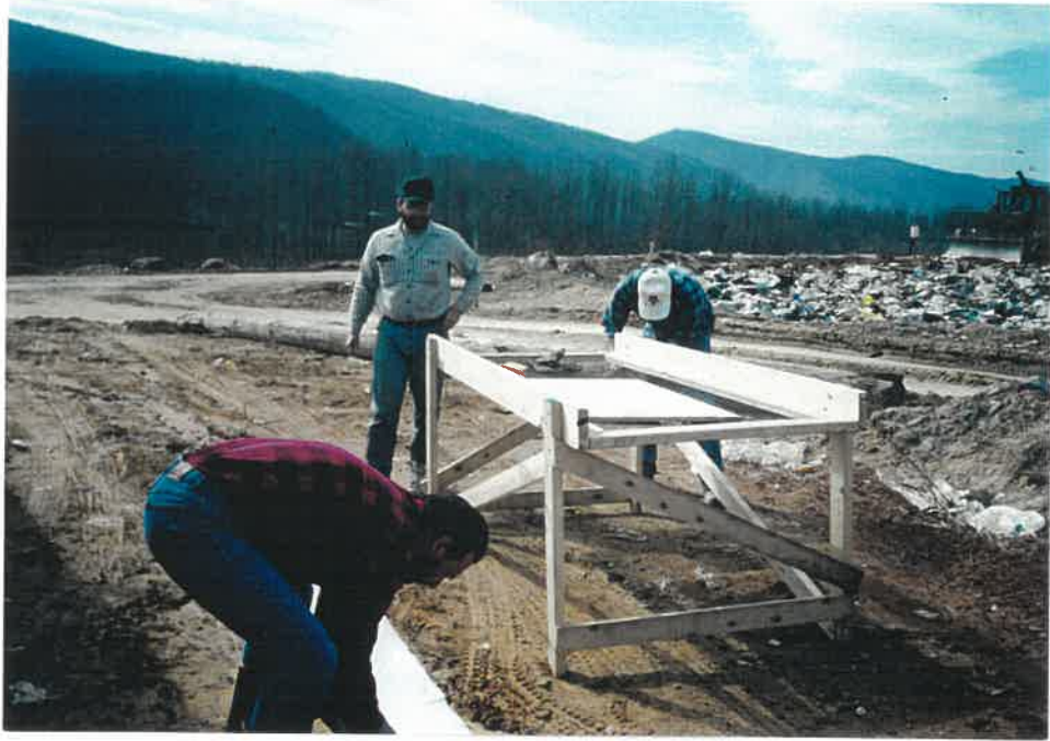
Photograph 3. Workers assembled the sorting table.
